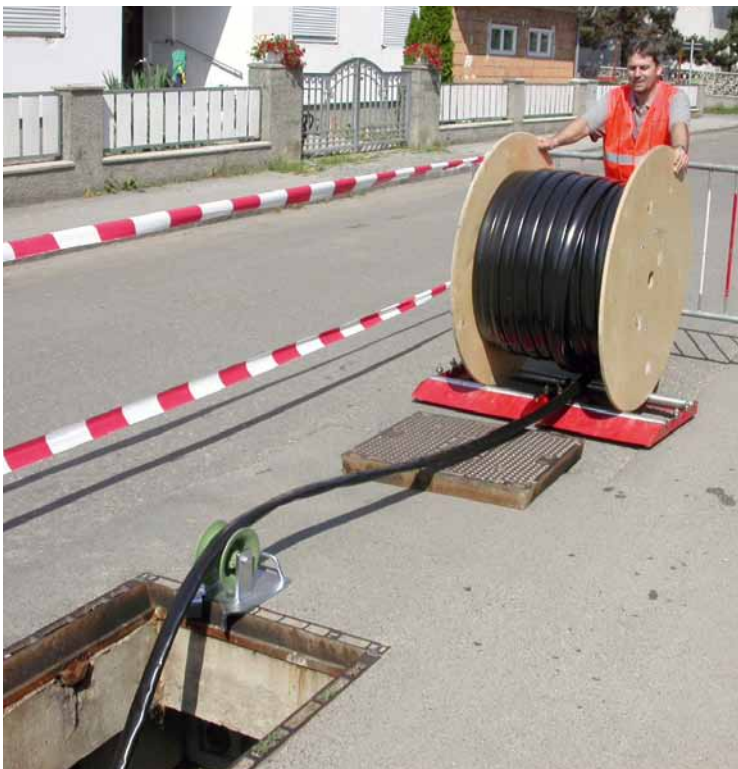
A speed•pipe® bundle SRV 50 / 8×10 is pulled into an existing PVC duct 110.
