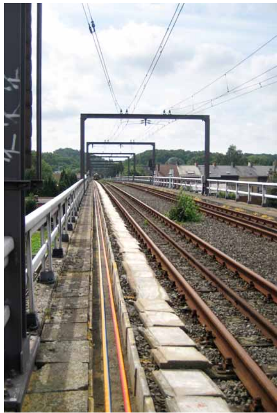
This picture illustrates a speed•pipe® bundle ground that was laid in a vat next to a railroad track.
