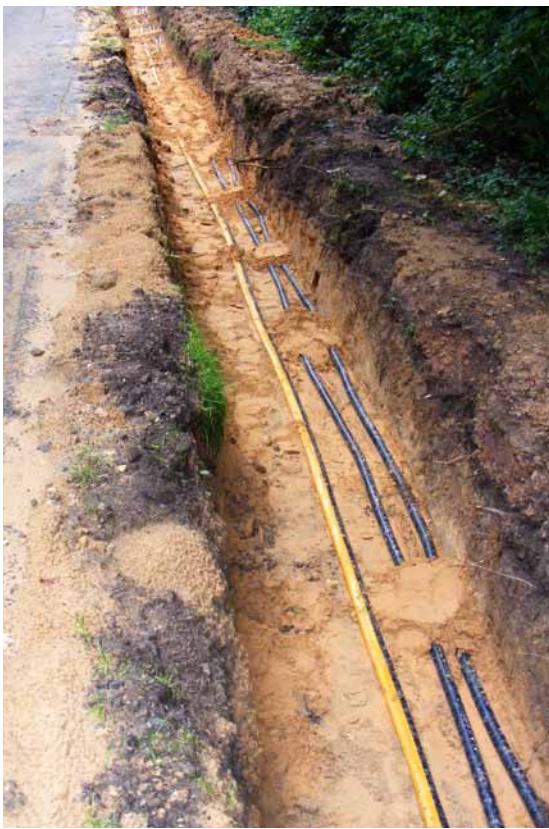
That is how the laying of the speed•pipe® bundle ground in an open trench looks like.
