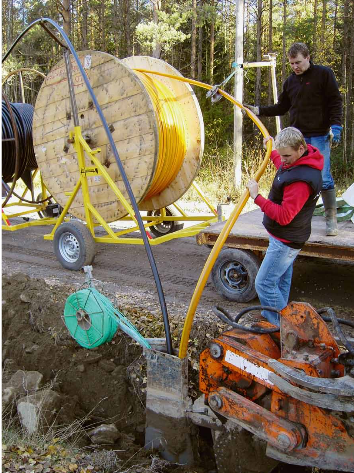
A speed•pipe® bundle ground is ploughed in.
