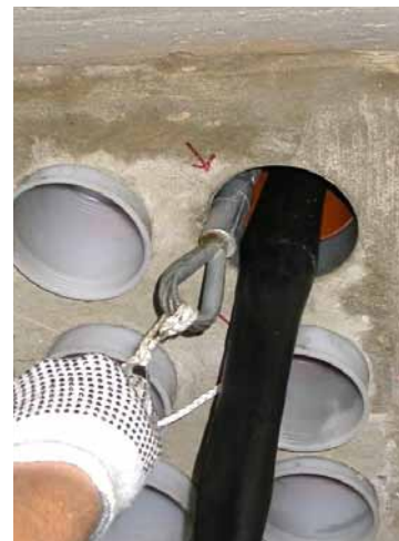
Here the PVC duct 110 is occupied with a second speed•pipe® bundle SRV 50 / 8×10.
